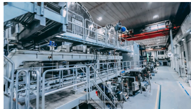
Metsä has started up the upgrades BM at the Simpele mill
