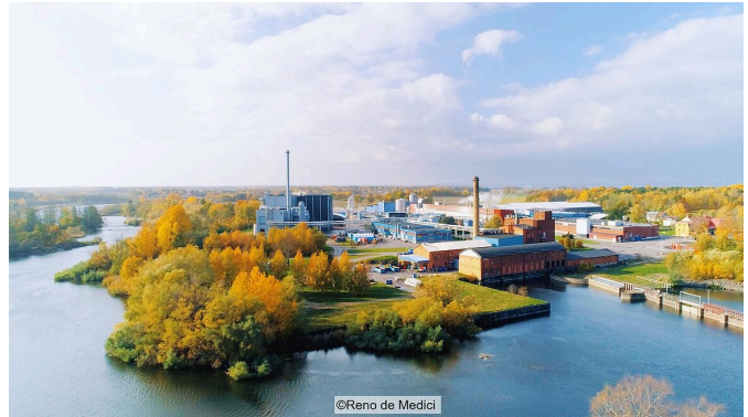
RDM operates eight mills in Europe, among them the Fiskeby facility
