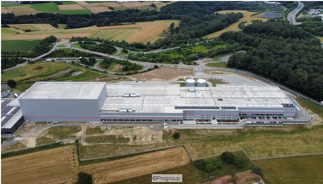
Progroup's new Petersberg plant
