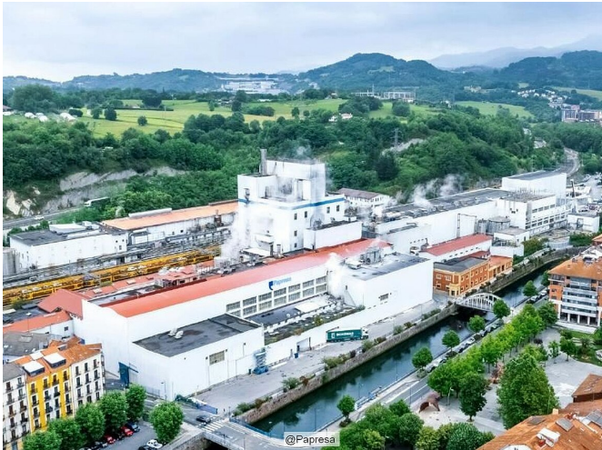
Papresa will install a Valmet Bale Tester
