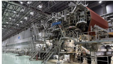
Aquakraft's PM2 containerboard mill in Ferizli, Turkey, will be upgraded by full-line supplier Voith through 2027.
